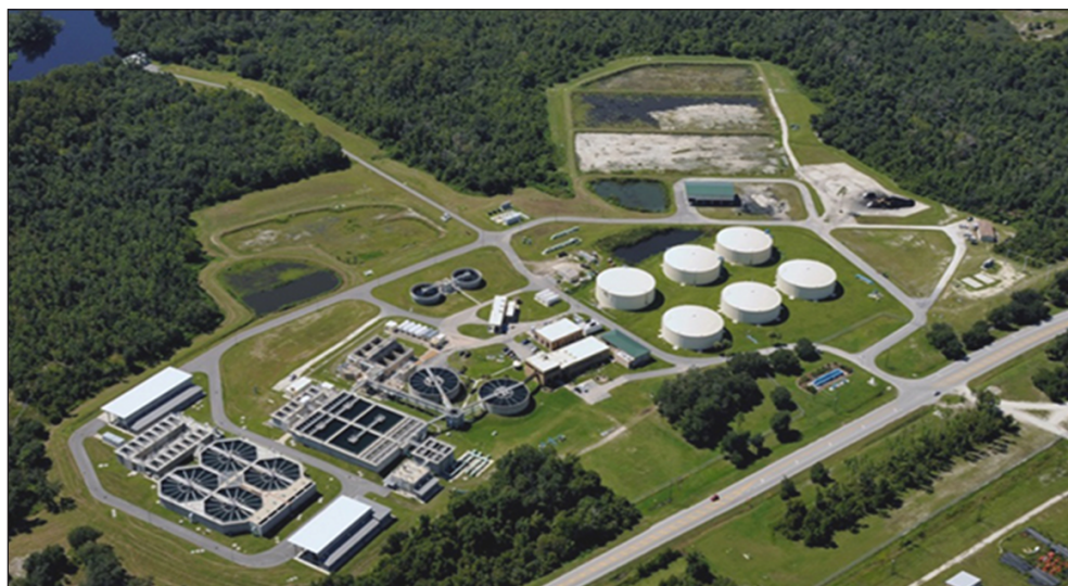
Figure 6. Peace River Manasota Regional Water Supply Authority Treatment Facility
